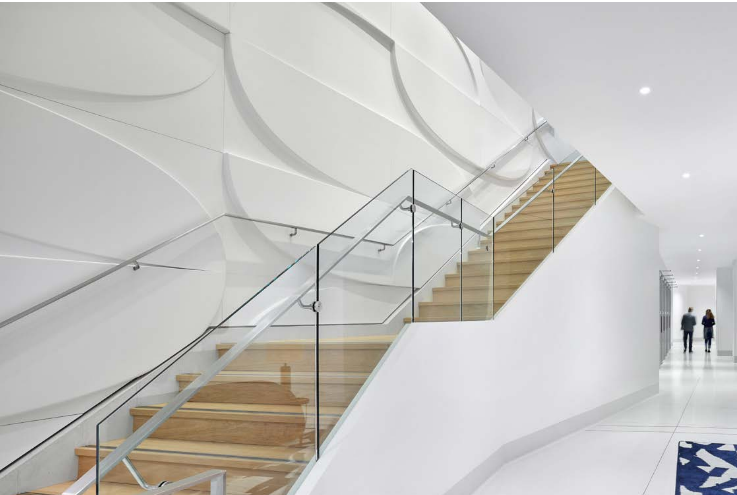
A custom CNC-cut pattern of fractured ovals based on the global environmental graphics pattern forms the 3-D MDF wall of the grand hall stair
